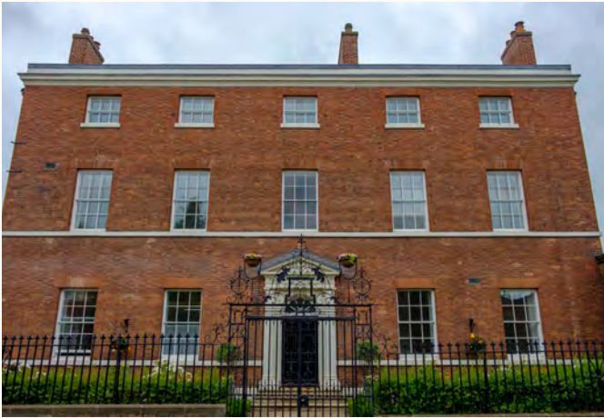
A typical arrangement of sash windows (note the vertical orientation of window lights on ground and first floor, and landscape orientation on the attic storey).
