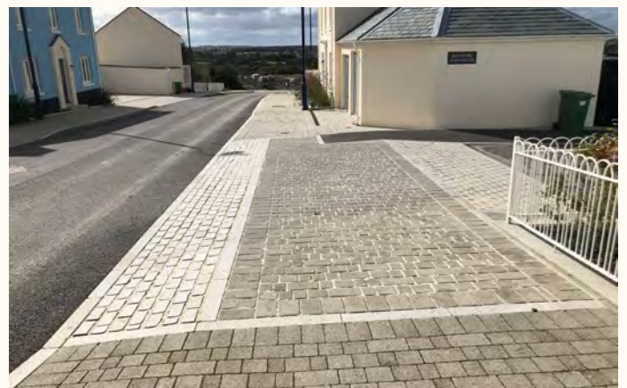
Example of a continuous crossing in Nansledan, Cornwall.
