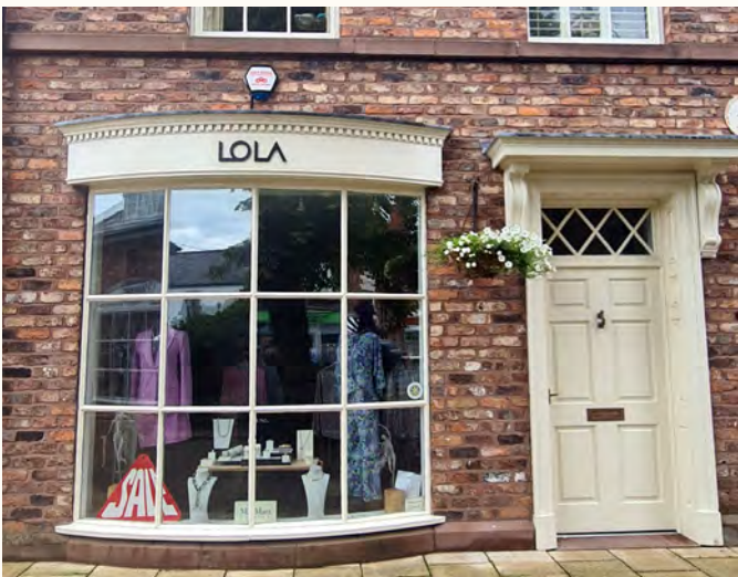
Example of simple vernacular mixed-use buildings (built 1993) in a sensitive historic setting, Tarporley, Cheshire.
